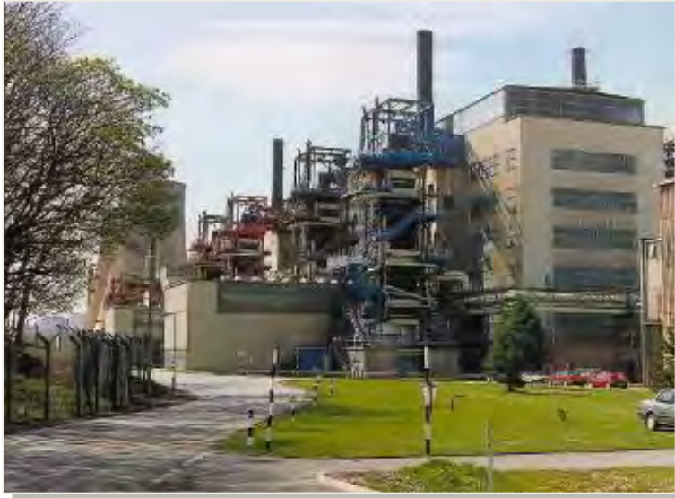
Magnox - Calder Hall
